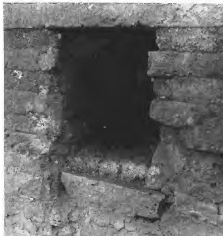
Fig. 192 b . S. Pietro in Vincoli, North clerestorey, beam hole for aisle roof, church A
